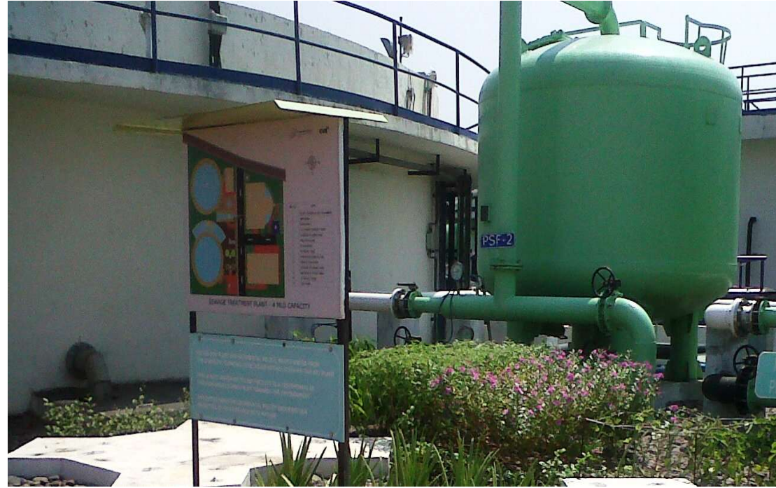
Sequential Batch Reactor & PSF
