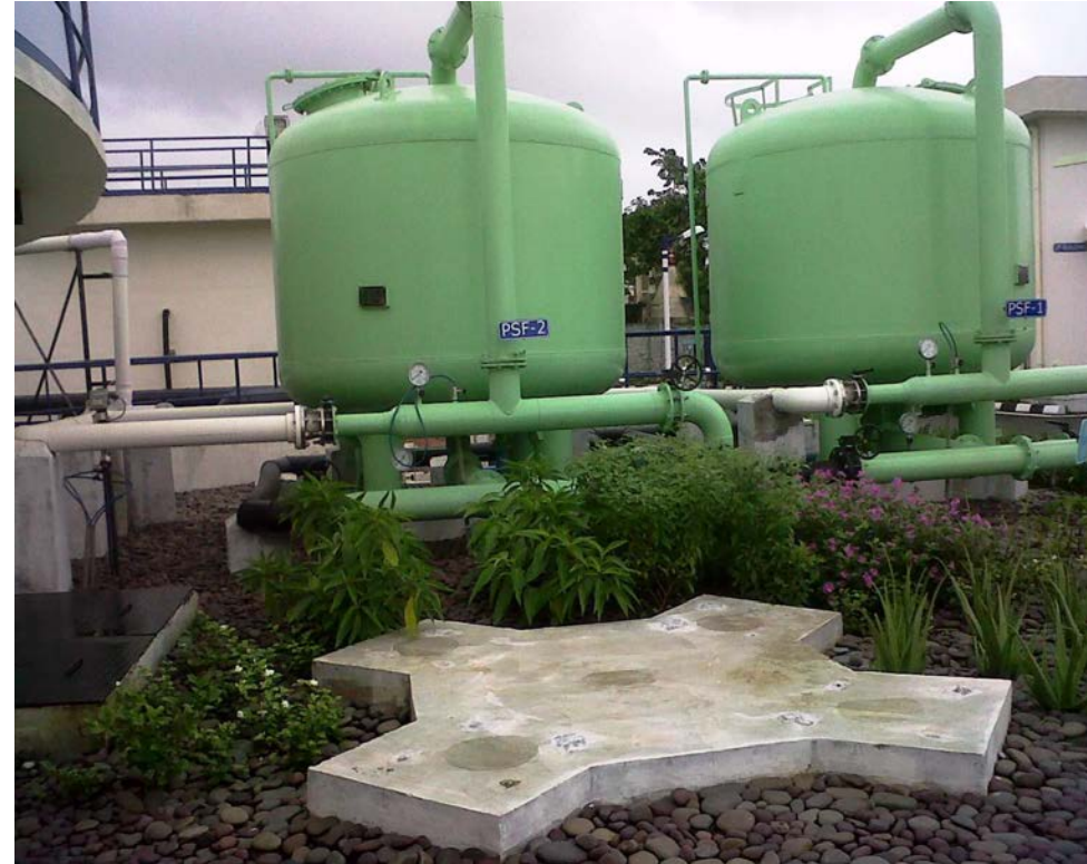
Pressure Sand Filters
